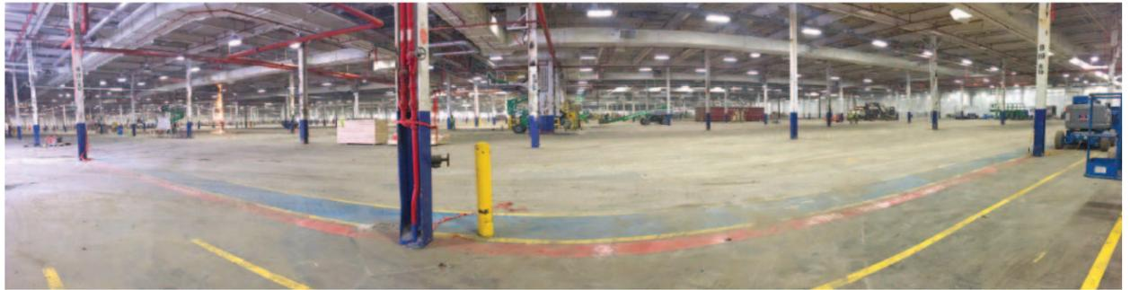
This new project began in early January and involved approximately 2.5 million square feet of floor space. Working two 10-hour shifts a day, seven days a week, the efforts continued into April. Approximately 9,200 gross tons of unprepared plate and structural and sheet iron along with over 1.35 million pounds of non-ferrous material were removed from the worksite.
